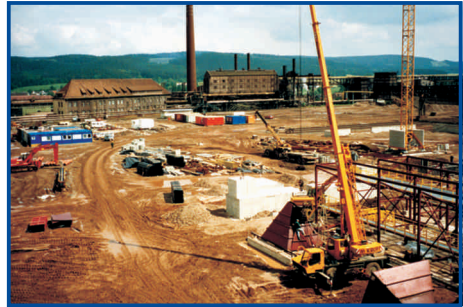
Construction of the electric steel plant
