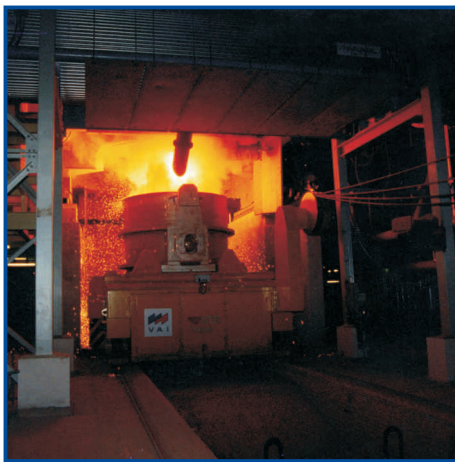
Tapping of the electric arc furnace
