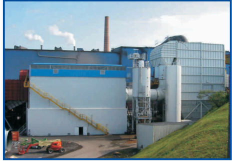
The de-dusting plant of the melting shop
